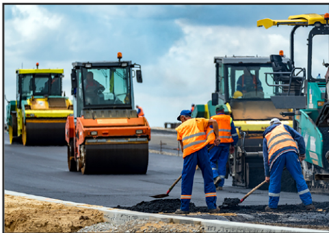
Highway Construction & Maintenance Crews
